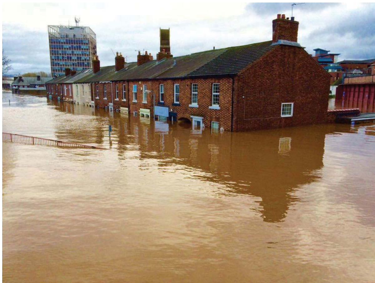
Figure 3: Illustration of the depths of water during Storm Desmond 2015 (Carlisle)
